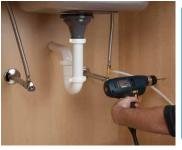
7 Use a 6mm drill bit to drill holes for the plastic anchors. Carefully tap the anchors into the drilled hole with a hammer. Mount unit to the wall with the screws. Pull the protective plastic strip from the battery compartment. The red LED should flash and beep five (5) times to indicate that the battery is installed correctly.
