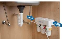
Connect supply lines: insert tubing from the tee fitting into the inlet side and insert tubing from the faucet into the outlet side. Use diagram on the right to mark tubing depth to ensure they get inserted completely. It is VERY IMPORTANT to insert tubing
