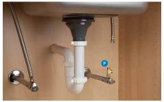
Attach threaded ends of supplied brass tee to the cold water supply line and shut-off valve; tighten using an adjustable wrench.
