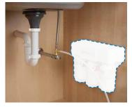
Unit Installation: Select a space under your sink for the filter unit that is at least 30cm from the bottom of your cabinet and allows for easy access to your cold water supply and for filter replacements. Use the mounting holes located at the back of the unit to mark the wall screw placements with a pencil. Center to center hole distance: 98mm.
