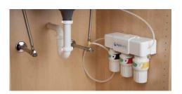
Turn the cold water on. Check for leaks and proper installation: place a towel under the filter unit and check for leaks. Allow water to run for 10 minutes to flush carbon fines.
